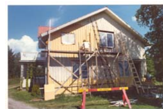
Repainting the house
